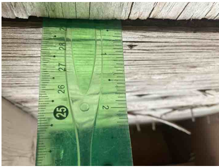
1/2 inch thick sheathing
